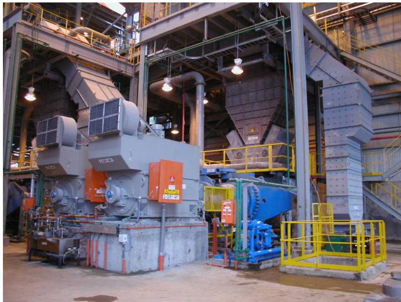
PT Freeport Indonesia's HPGRs with feed and by-pass chutes
